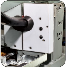
扶手带出入口保护装置 Handrail entry and exit guard
