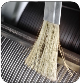
扶梯导静电装置 Handrail anti-static device
