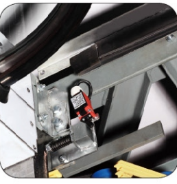
梳齿保护 Comb plate safety device
